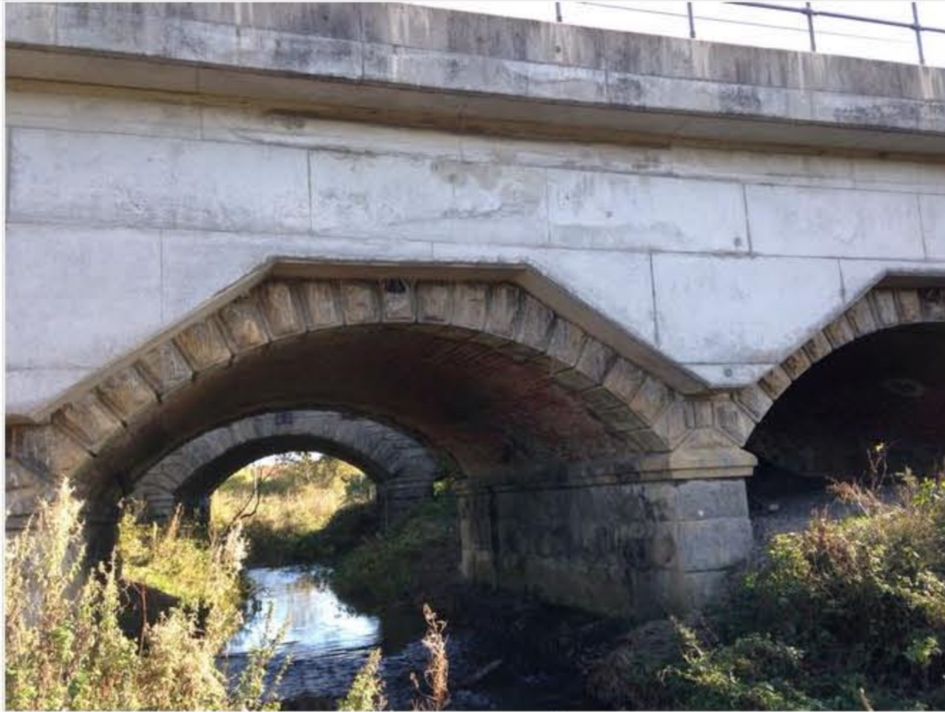
One of this weeks scour protection surveys
