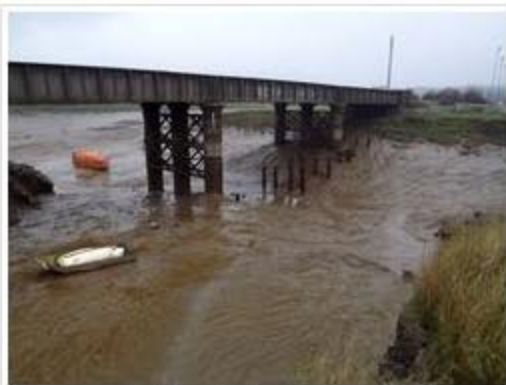
One of the bridges on a tidal inlet
