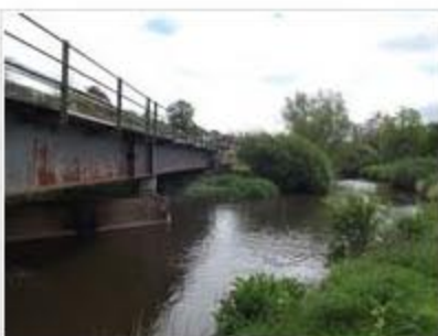
Railway bridge deck survey
