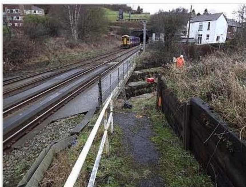
Scour protection survey to protect railway bridge
